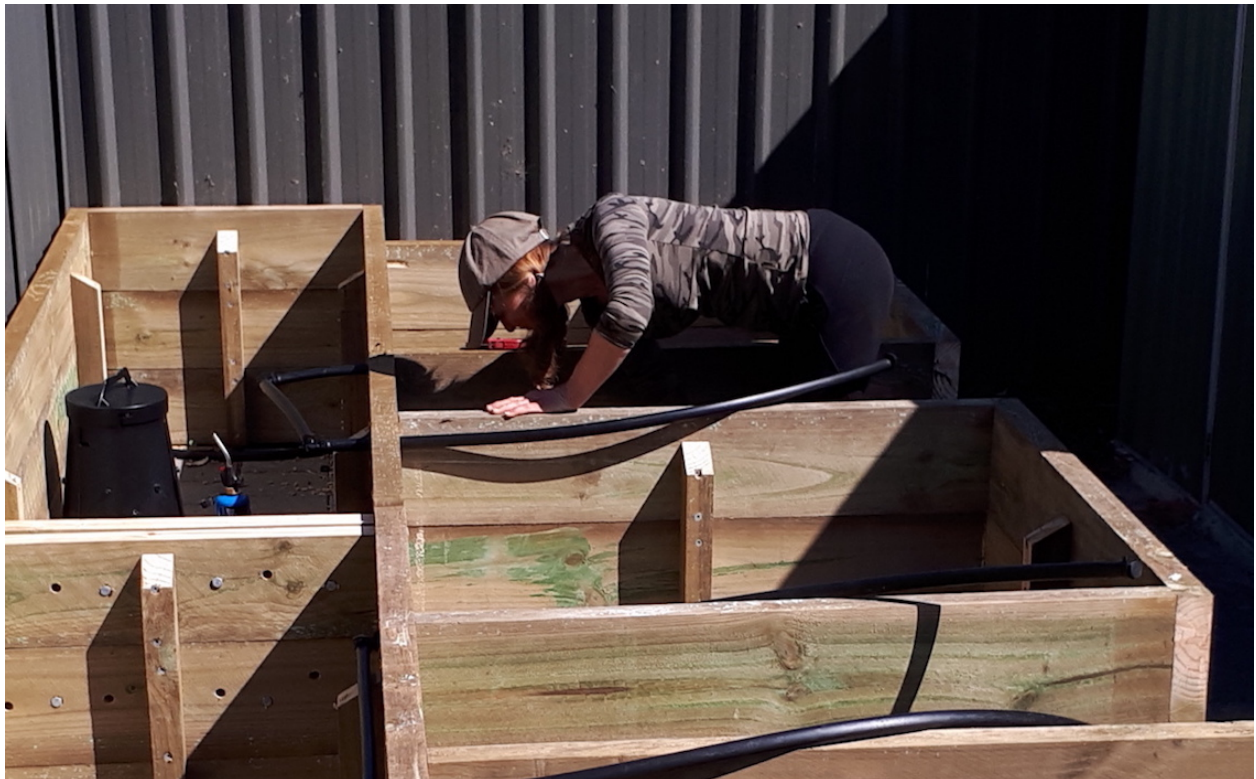
Threading irrigation pipe through holes drilled into the beds.
